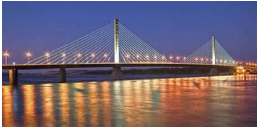
Aswan Bridge Loading Test
