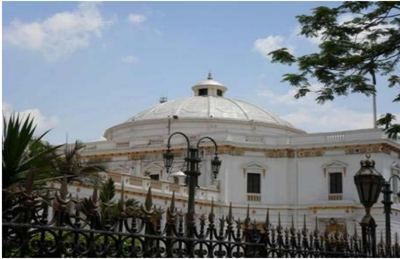
Design and Supervision of Repair Works of Parliament Building
