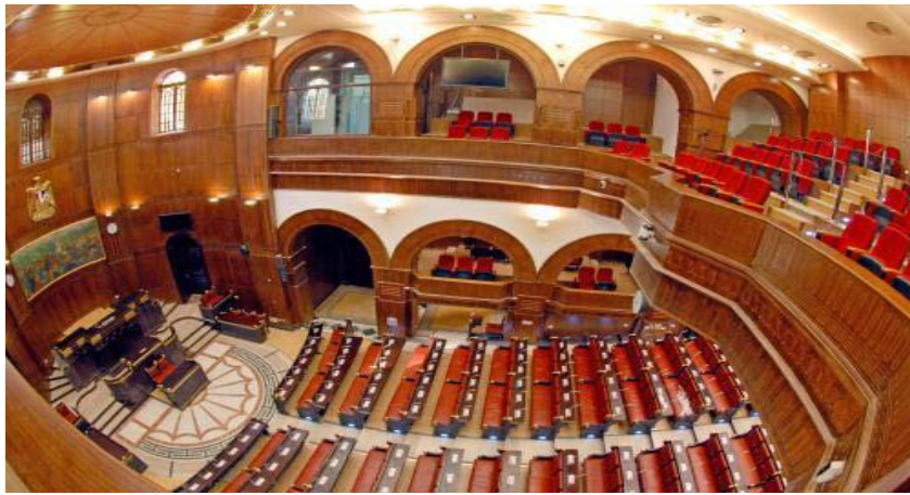
Design and Supervision of Repair Works of Shoura Building
