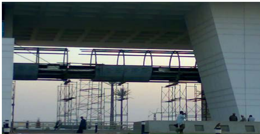
Pedestrian Bridge Loading Test
