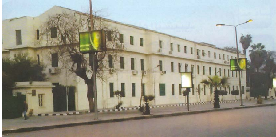
Materials Testing Laboratory Overlooking El-Jamaa Street
